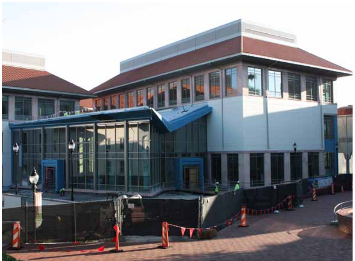
Construction still under way with blue waterproofing yet to be covered.
